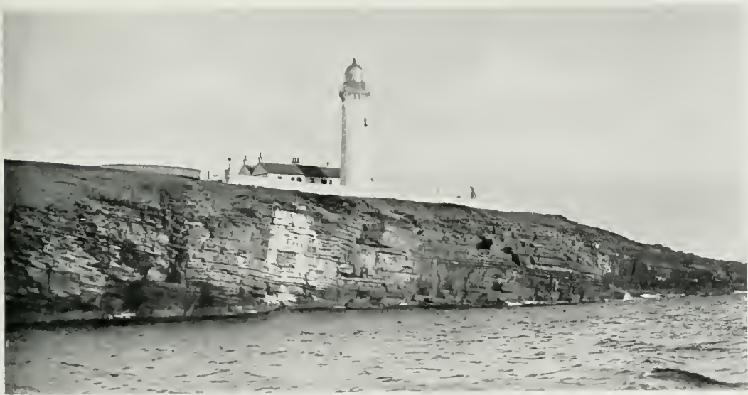
CANTICK LIGHTHOUSE, SOUTH WALLS.
